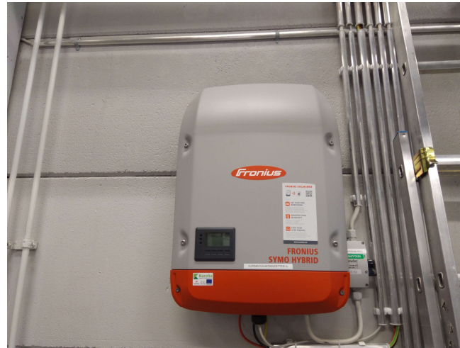
Fronius Symo Hybrid 5 kW
